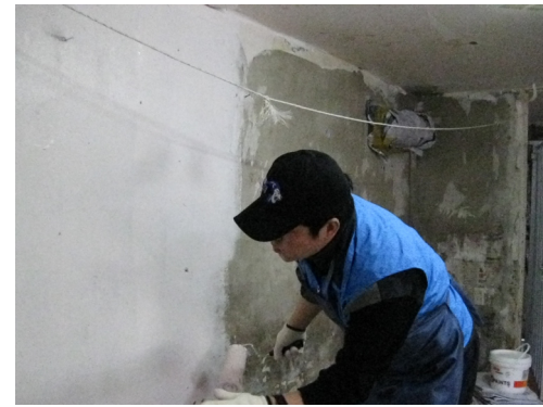
A volunteer paints the walls in Daejeon Shelter
